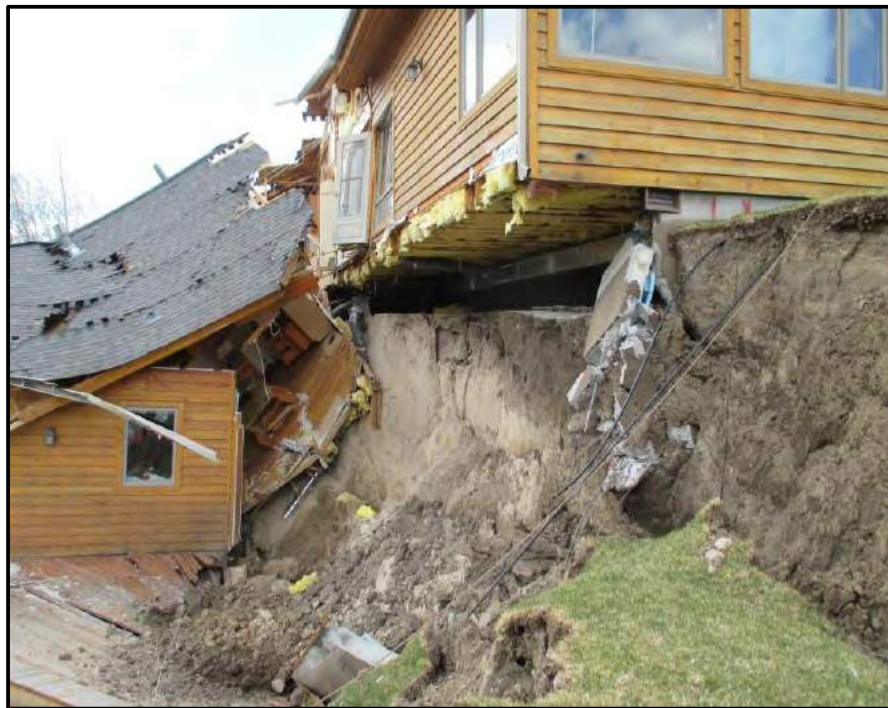
Figure 20: Headscarp of the landslide directly under the inside edge of the southeastern foundation of the house at 1045 Budge Drive
