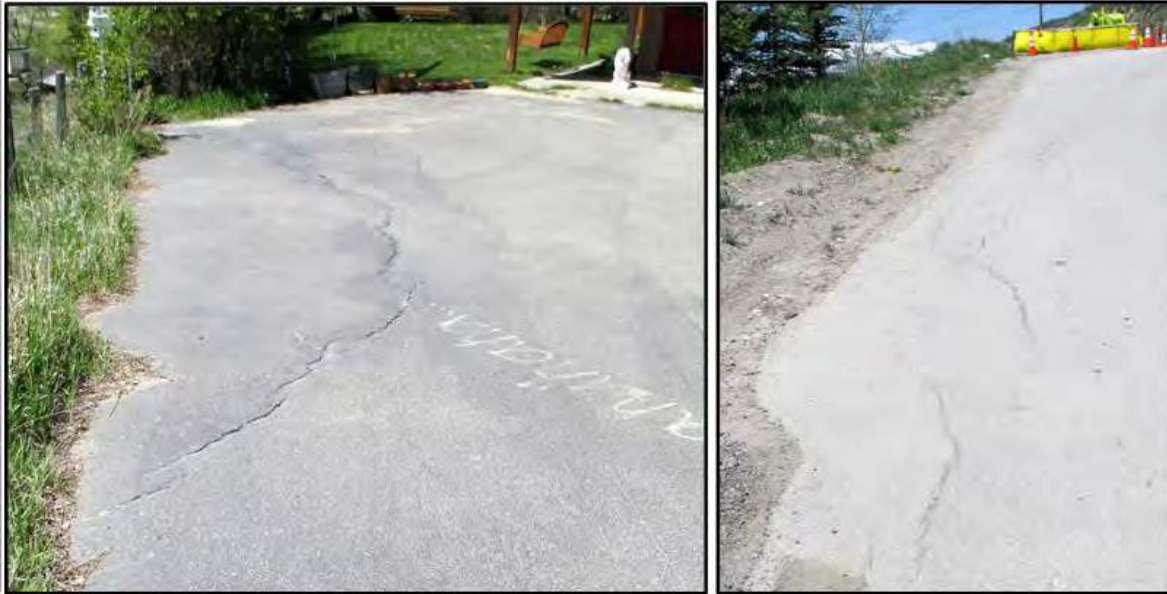
Figure 15: Crack in the driveway at 980 Budge Drive (left) and just to the north along Budge Drive (right) that were first observed in 2009 shortly after a malfunction of the sprinkler system for the condominiums at 981 Budge Drive caused considerable water to flow down the hill. Views looking west.
