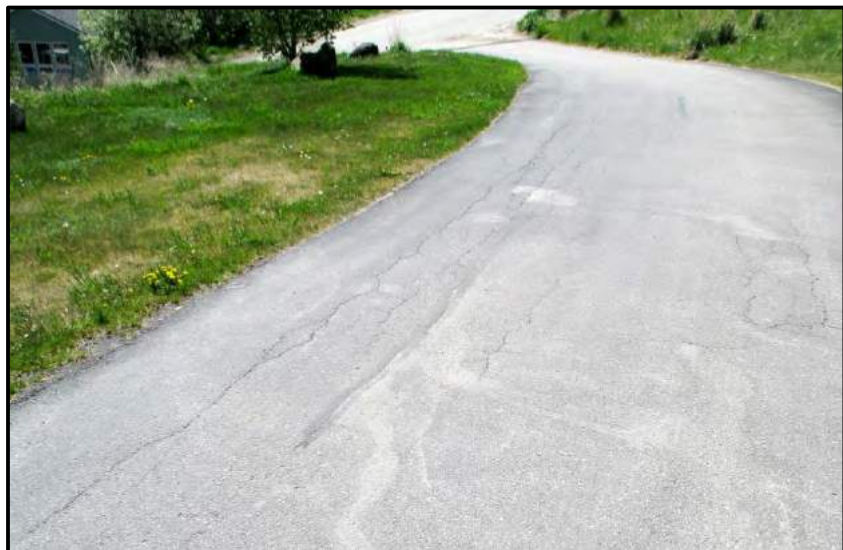
Figure 16: Cracks in the driveway to the condominiums at 981 Budge Drive, looking west.
