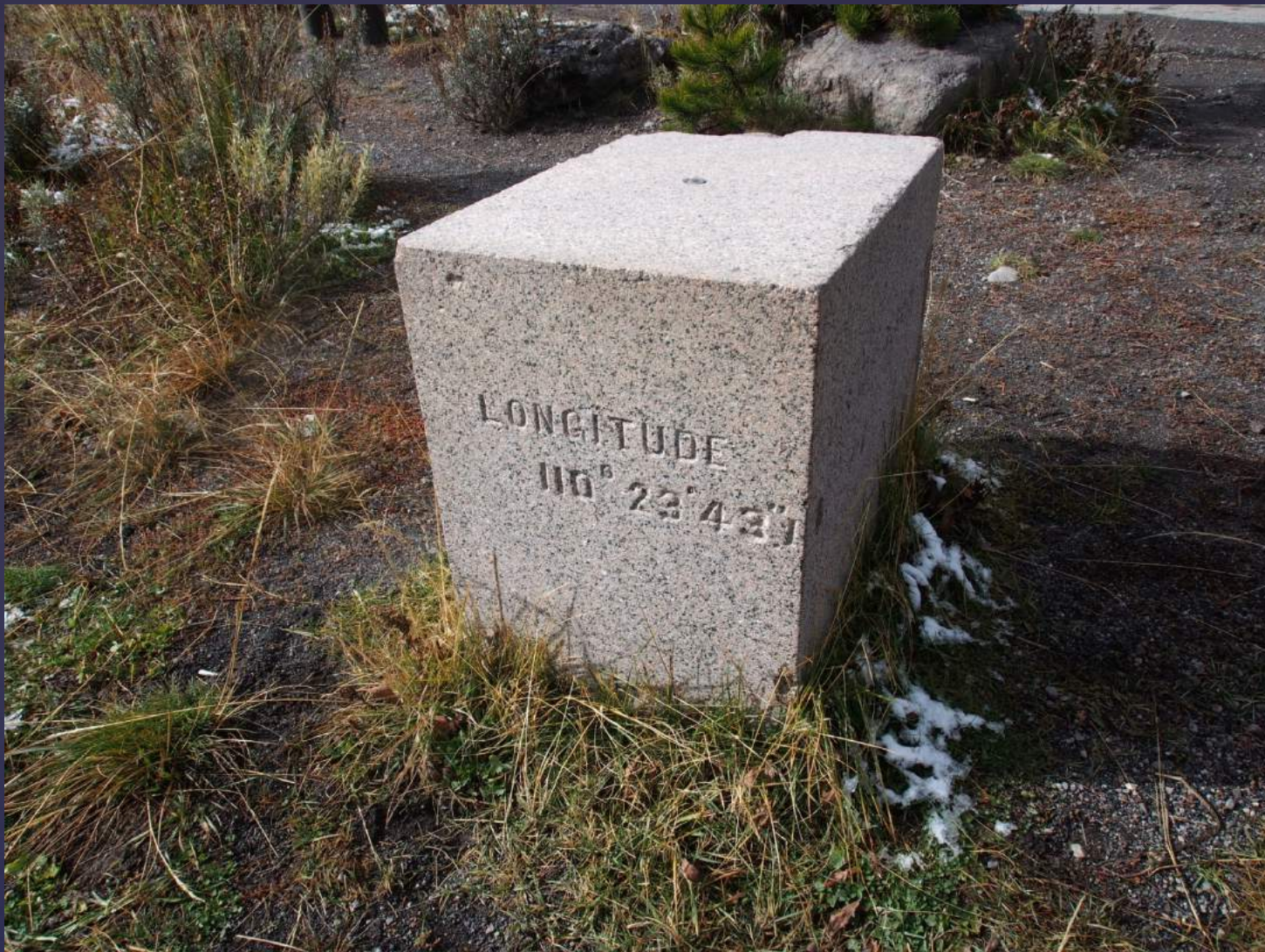
Lake Astro Station, Yellowstone NP, U.S. Coast and Geodetic Survey, C.H. Sinclair and G.R. Putnam, May 30 to June 30 1892. T.M. Bannon included this station in his triangulation network as a latitude-longitude check.
